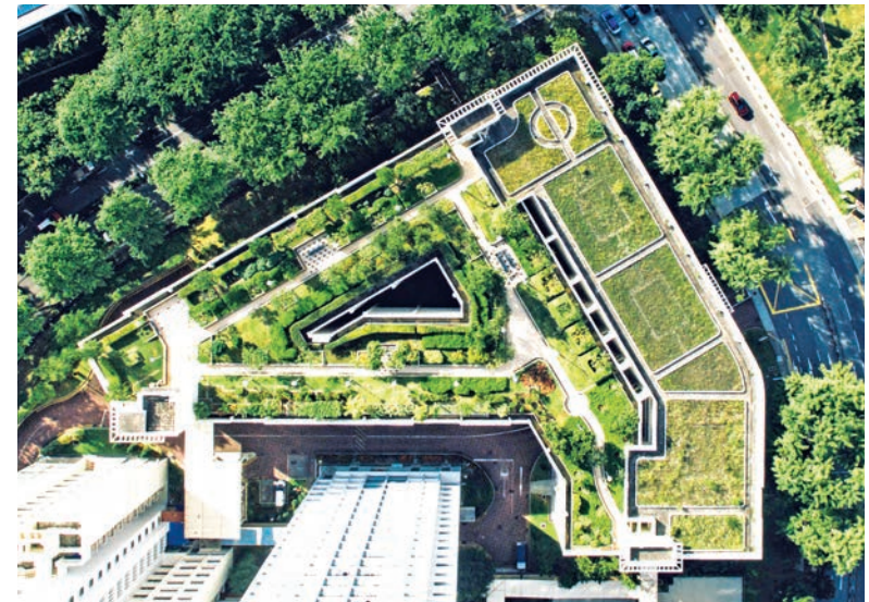
17. Rooftop gardens connect residential blocks for convenience and accessibility and encourage outdoor activity.
