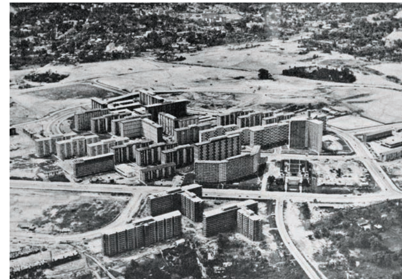
15. Aerial view of Toa Payoh in 1967. Its town centre was a focal point where residents could meet and shop.
