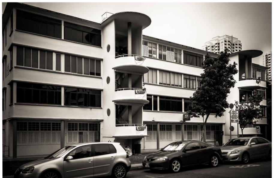
Old apartment blocks in Tiong Bahru built by the Singapore Improvement Trust (SIT). SIT was the housing agency formed under the colonial government. It built some flats, but not enough to resolve a housing crisis that became increasingly severe under its watch. Source: Dickson Phua flickr.com/photos/gunman47/14649721988
