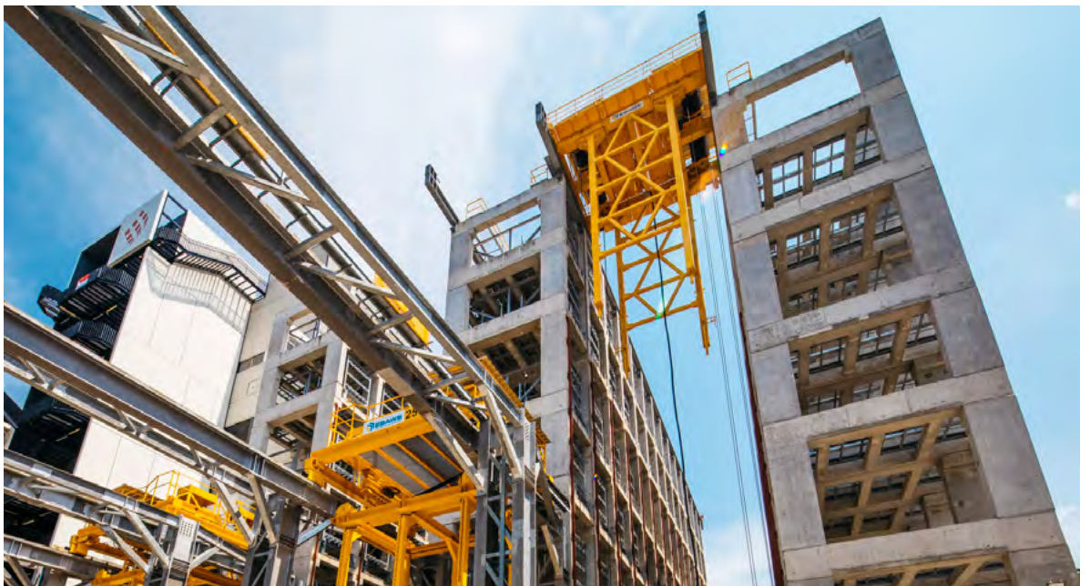
Fig 6. Straits Construction Group's Greyform Building, an example of an Integrated Construction and Prefabrication Hub, a multi-storey manufacturing facility with a high degree of mechanisation and automation that allows for more efficient land and space utilisation.. Image courtesy of Straits Construction Group.
