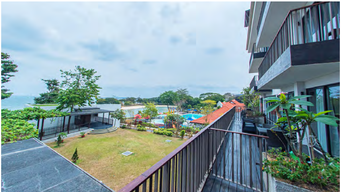
Fig 1. Since SARS, Singapore has increased its quarantine capacity, including preparing chalets as backup emergency housing, holding drill exercises and occasionally activating them. These were quickly activated when COVID-19 struck. Image courtesy of Civil Service College.
