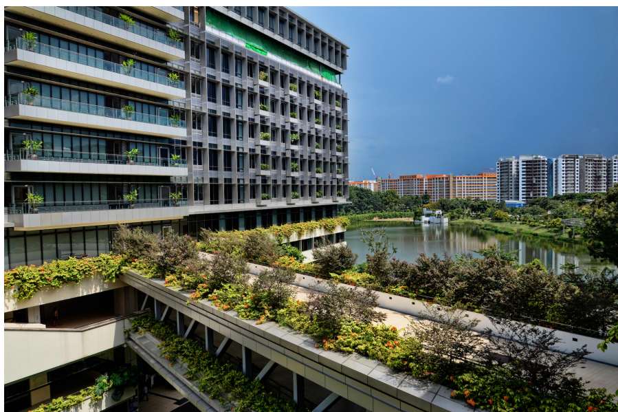
Figure 3: The public healthcare landscape is structured into three clusters, each encompassing a full range of services. Khoo Teck Puat Hospital is part of the Central cluster, sited within a HDB neighbourhood and is highly accessible to the residents. Source: William Cho
