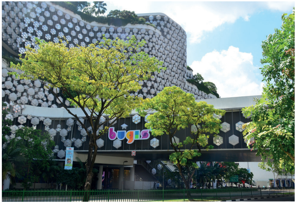
Bugis+ (formerly Iluma) is the outcome of a government land sale at Victoria Street in 2005, where developers could tender for either a 30 year or 60 year lease. Image credit: Choo Yut Shing @ https://flic.kr/p/chUAUu
