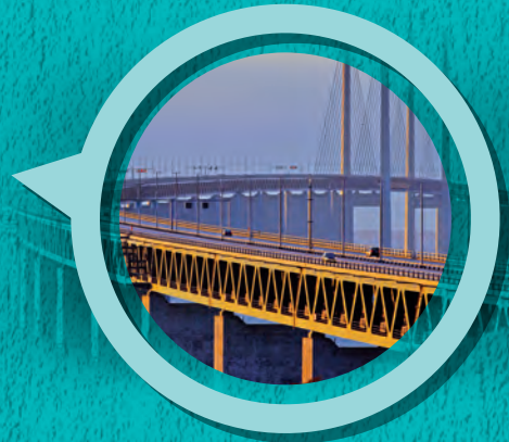
12 The Øresund Bridge Linking Copenhagen, Denmark and Malmö, Sweden together, the bridge symbolises aggregation of a greater economic base for revitalisation of the city’s economy.
