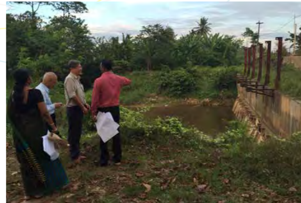
Sri Lankan officials explaining the operation of the weir upstream of the Thalangama Tank, as part of the Madiwela East Diversion Scheme for flood management.
